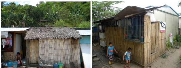
Figure 6: Precarious extensions in Village 2, using nipa leaves, wood and bamboo (left), and combined bamboo for walls and corrugated galvanized steel sheets for roofing (right).
